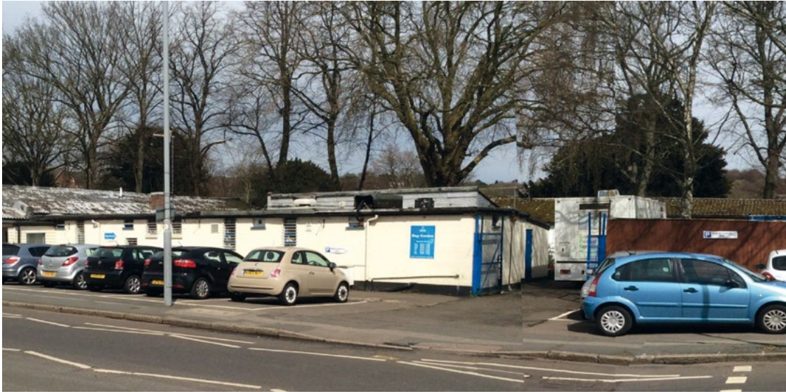
The Current Welfare Centre in Park Street, Luton
